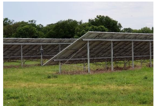
Example of a Solar Conversion System, Ground-mounted
