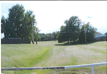
An Example of Stormwater Management An Example of Stormwater Retention
