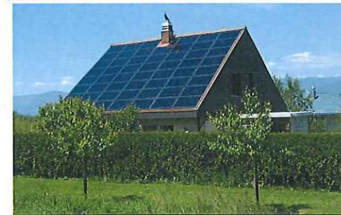
Example of a Solar Conversion System, Structure-mounted
