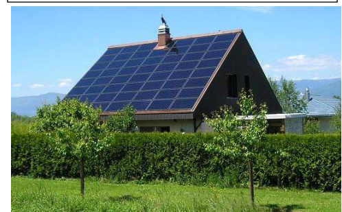
Example of a Solar Conversion System, Structure-mounted
