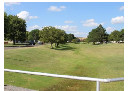
Example of a Drainageway
