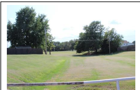
An Example of Stormwater Management An Example of Stormwater Retention
